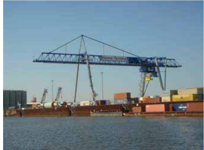
Harbor crane system
