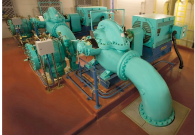
Boiler feed pumps
