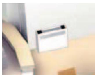
**11** - The convectors are automatically regulated by the **AT** time switch according to the program selected.
