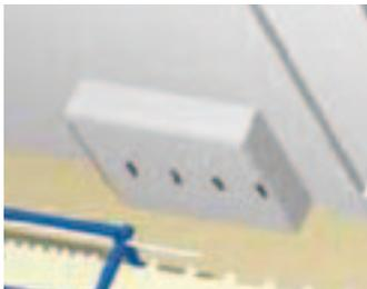
**1** - The temperature in the switchboards is controlled by the **THS-S**, which maintains it at the selected setpoint.
