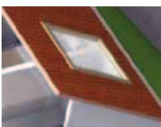
**6** - The skylight can be opened and closed to suit requirements by digital time switch **D1**, or by the **TW2/10K** twilight switch for daytime applications.
