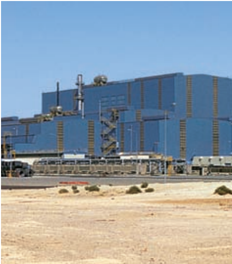
Turnkey package solutions: Large-scale projects for Hadeed
