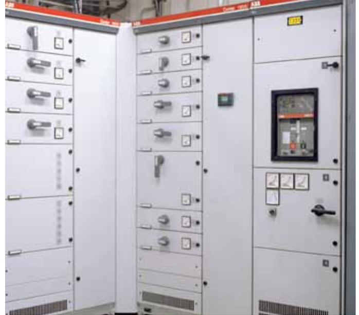
Arc Guard System™ — TVOC-2 installed in an ABB Low Voltage Switchgear
